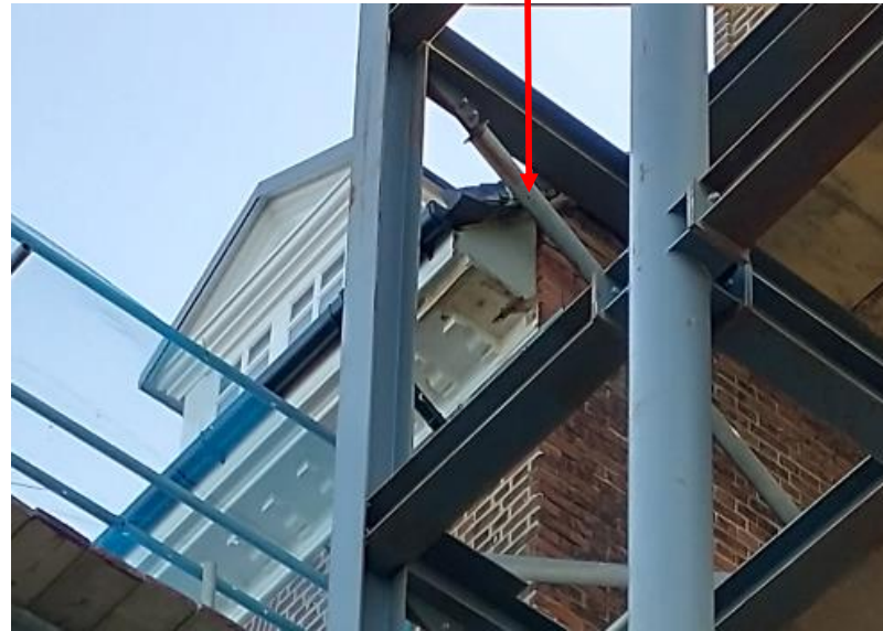
Eaves and cornice detailing removed
